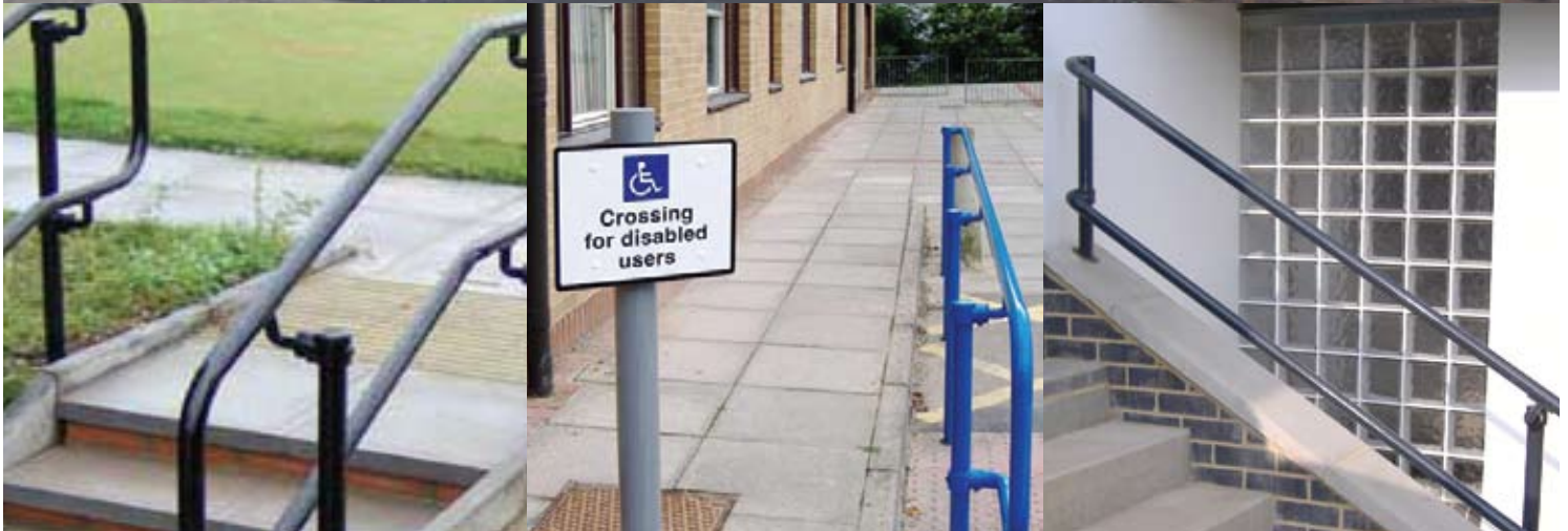
Mid rail comprises standard Kee Klamp® fittings
